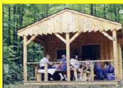
Pine Lodge Sleeps 6 Electric, "Inside Outhouse" (sink & flush toilet)
